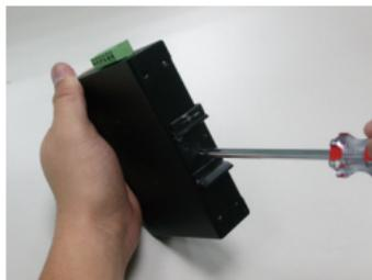
**Step 1:** Screw the DIN-rail bracket on the Industrial Media Converter.
